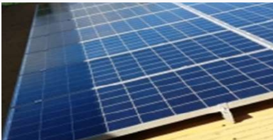
Figure 49: Building gets constructed near your mounting structure
