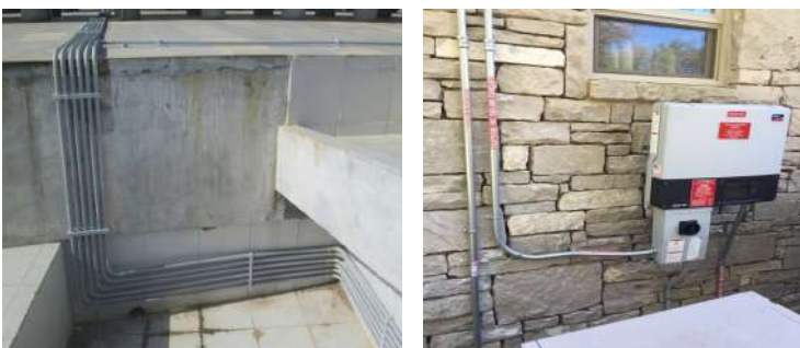
Figure 101: Proper cable routing
