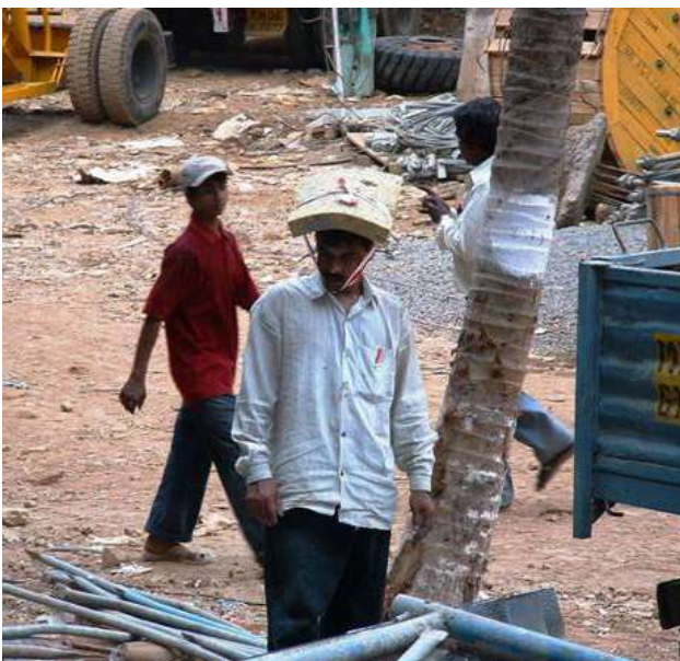
Figure 150: Incorrect practice - Without safety helmet
