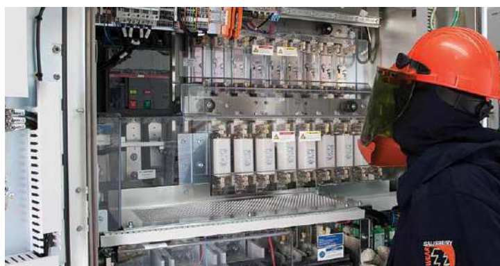
Figure 92: Check inverter fuses
