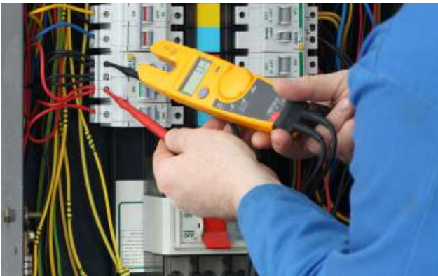
Figure 158: Incorrect practice - Without safety gloves
