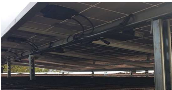
Figure 104: Correct cabling connection
