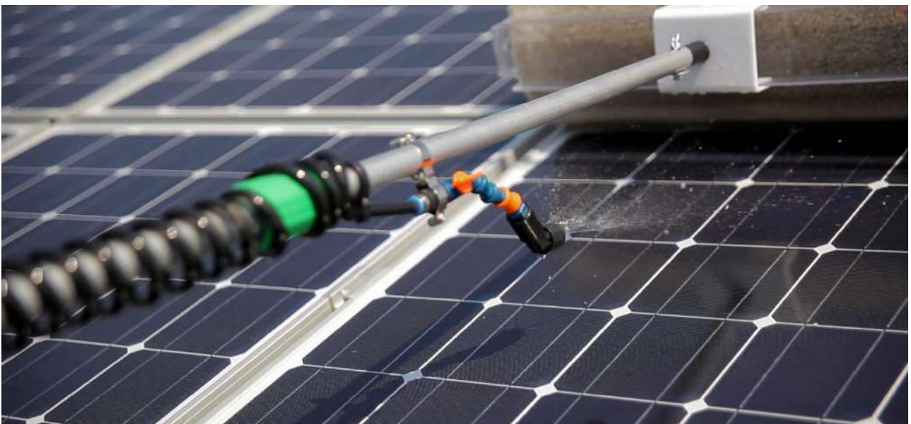
Figure 45: Wet cleaning using an automated system
