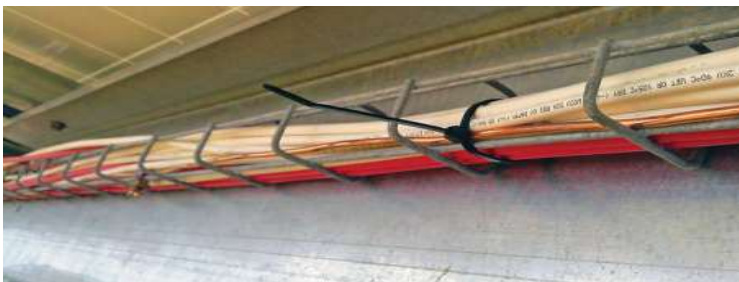
Figure 113: Cables are tied using cable tie
