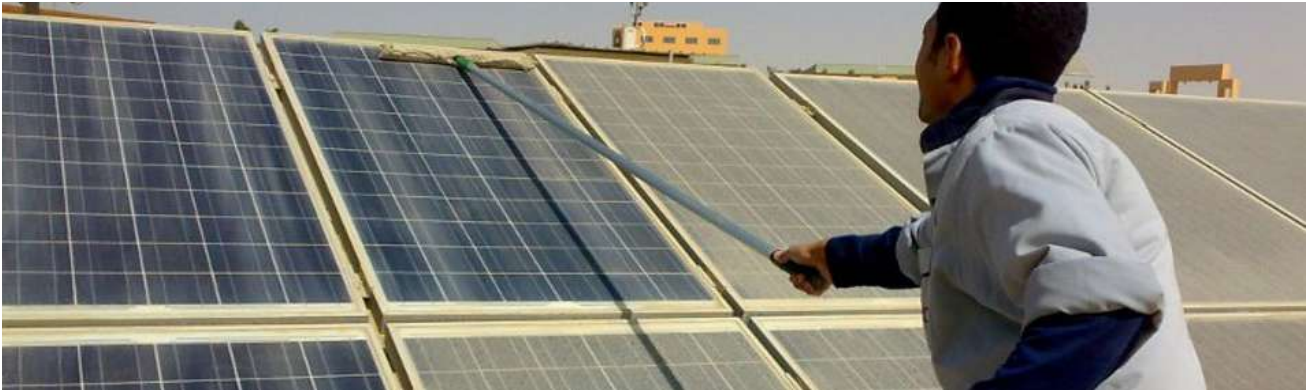
Figure 42: Dry Cleaning Method (Manual)
