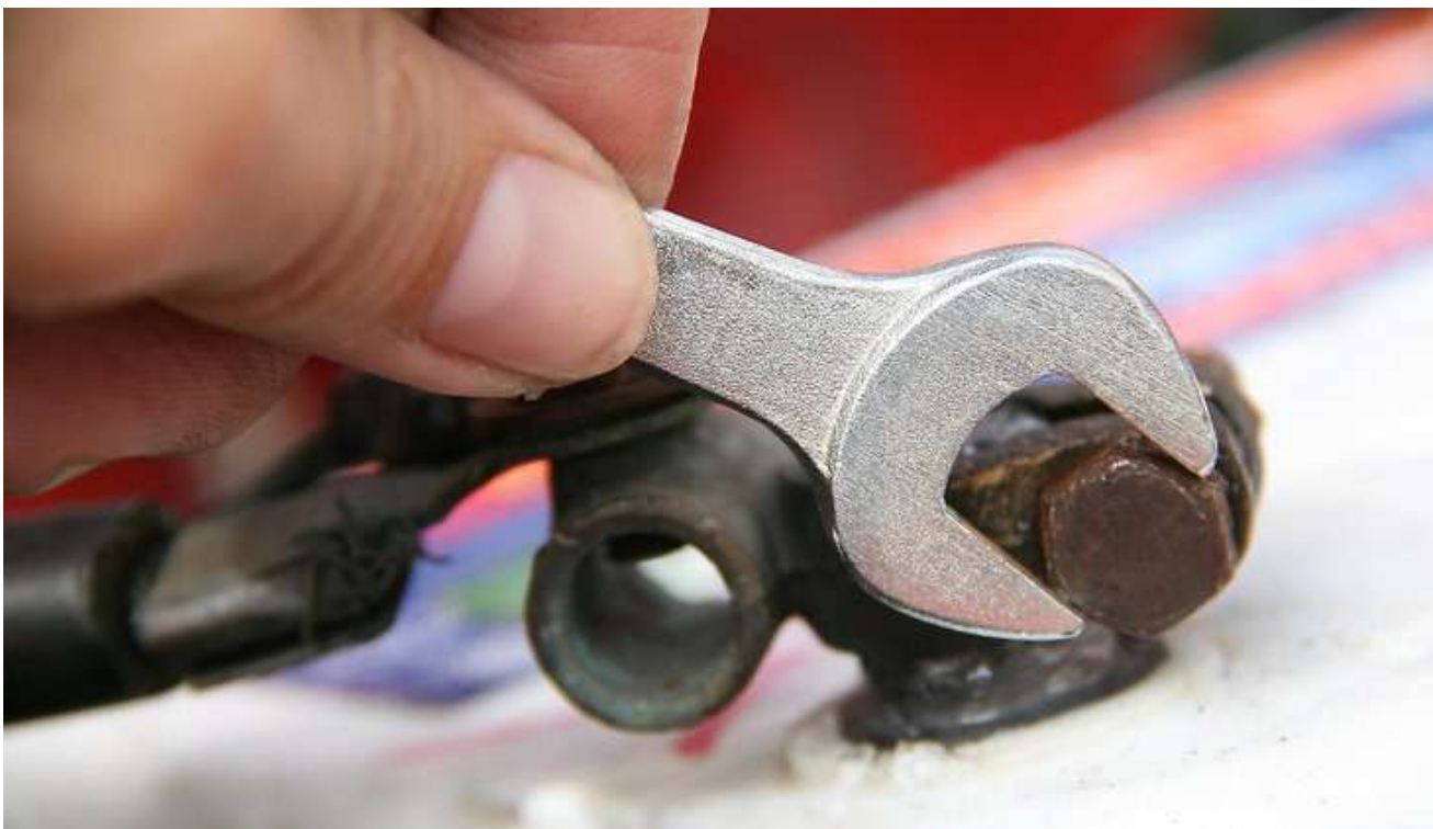
Figure 131: Tightened battery terminals
