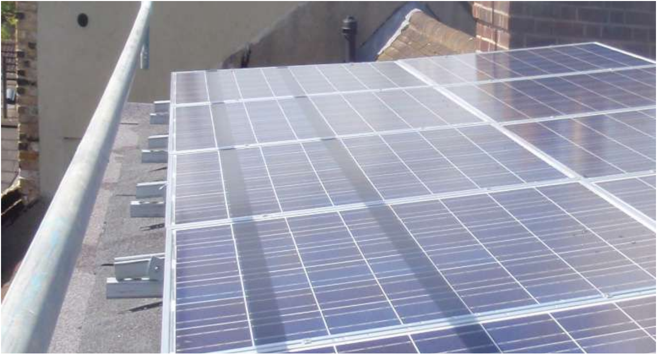
Figure 51: Shading due to nearby poles on terrace
