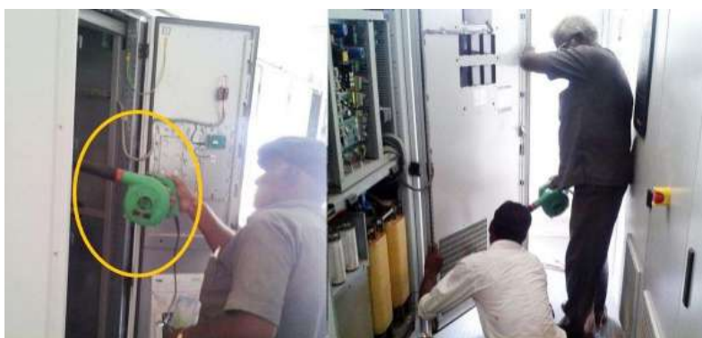
Figure 89: Cleaning inverter using blower
