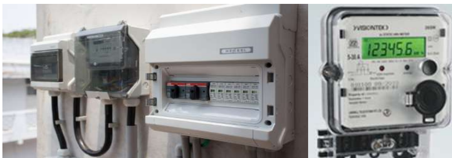
Figure 137: Net metering display screen showing units consumed by consumer
