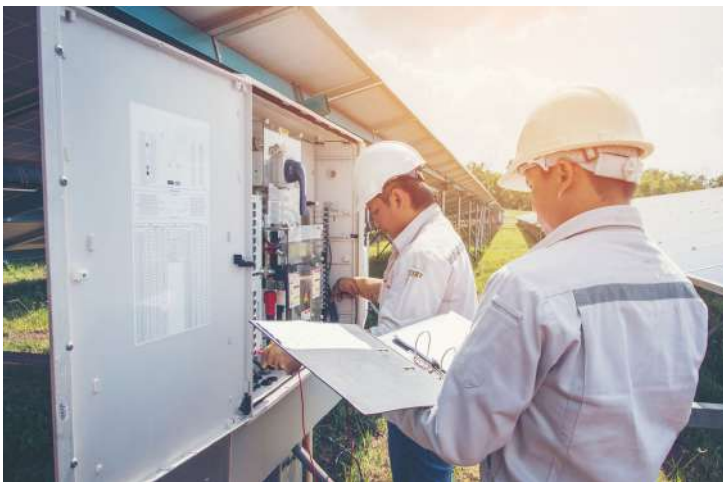
Figure 94: Written inspection report of Inverter
