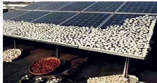
Figure 50: Shading due to drying crops
