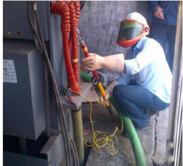
Figure 155: Correct practice - With face shield
