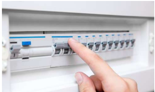
Figure 74: Switch off inverter before performing any maintenance
