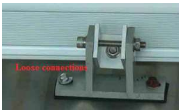
Figure 118: Loosed clamps
