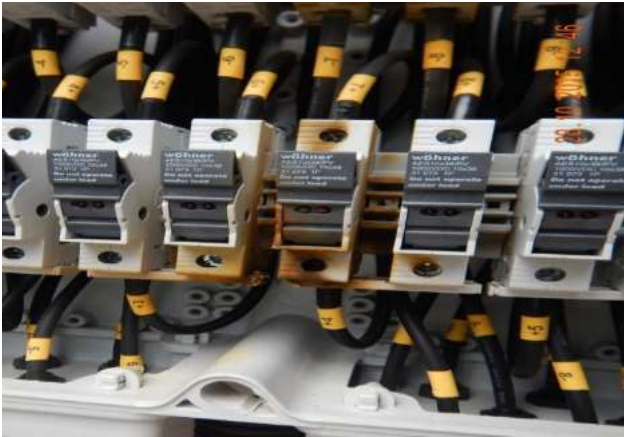
Figure 120: Fuses - Burnt out
