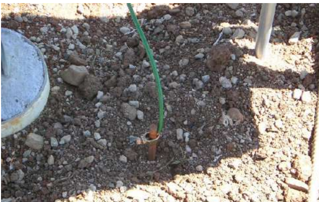
Figure 121: Grounding
