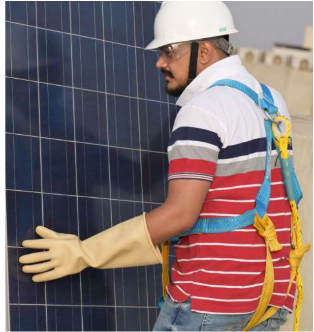
Figure 161: Correct practice - With safety belts
