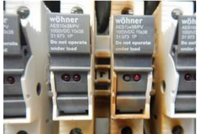
Figure 120: Fuses - Burnt out
