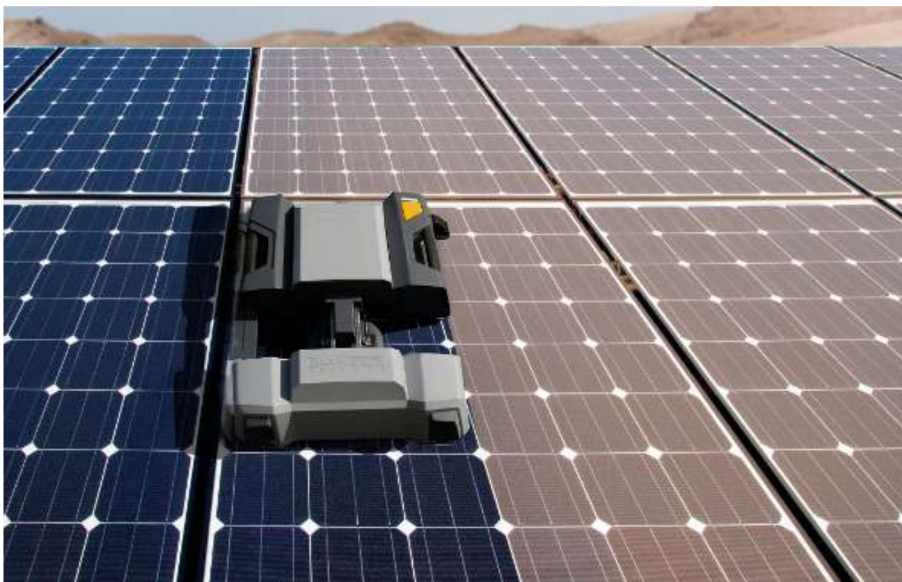
Figure 46: Dry cleaning method using an automated system
