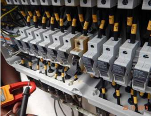
Figure140: Testing using clamp meter
