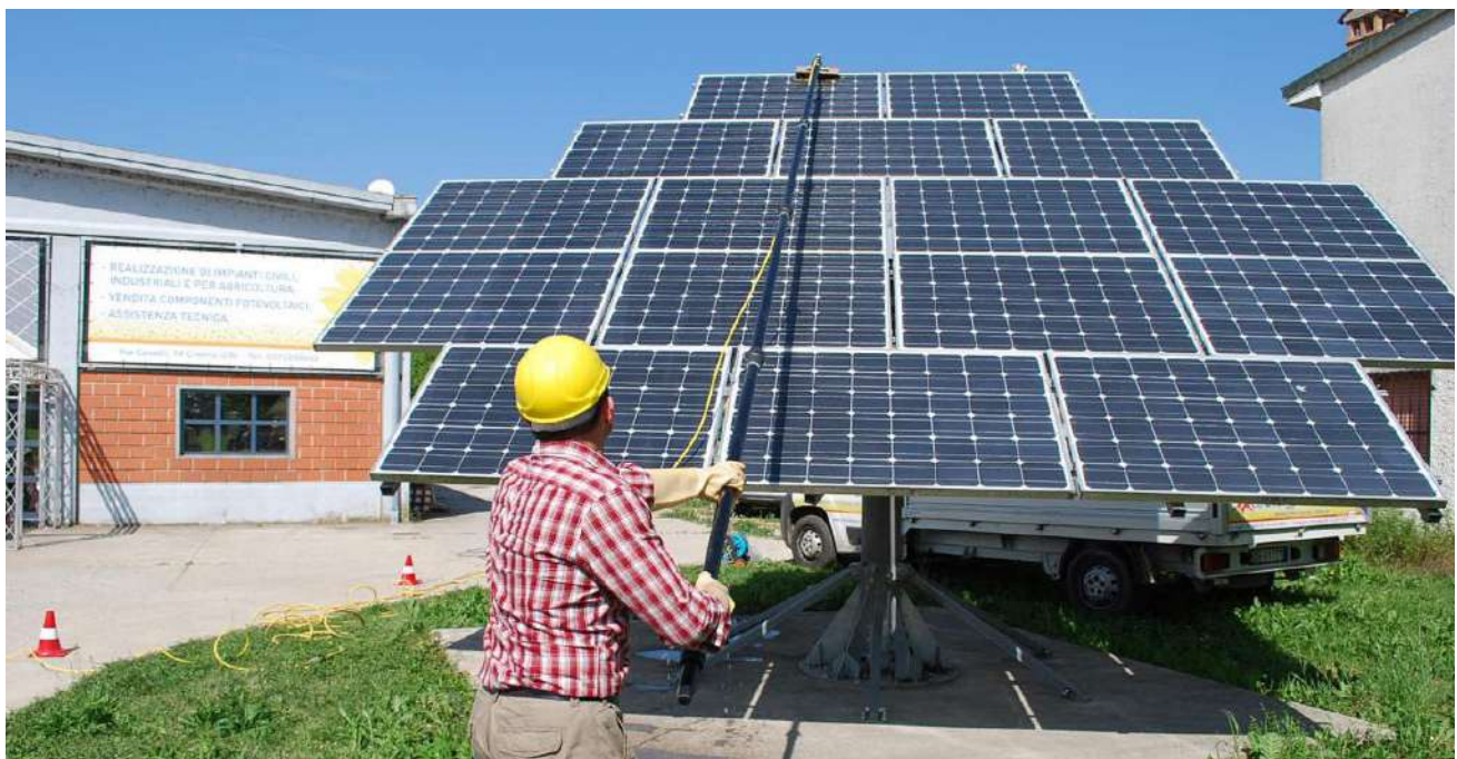
Figure 37: Wet Cleaning (Manual)
